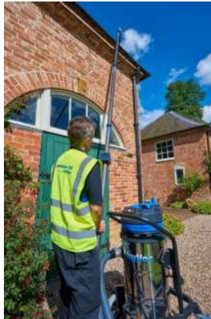
Fig 1 – gutter clearance using a vacuum
